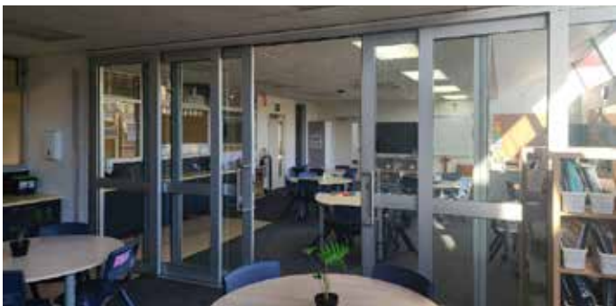
Installation of glass partition doors between Rooms 9 and 10
