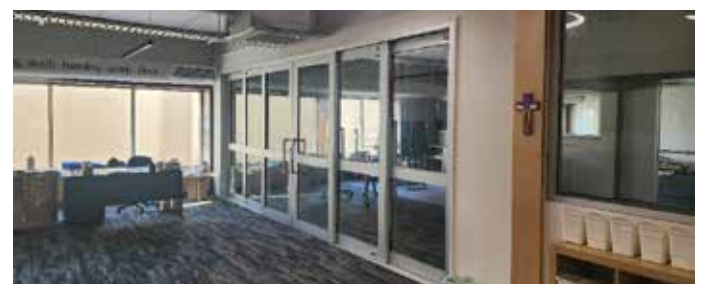
Installation of glass partition doors between Rooms 12A & 12B
