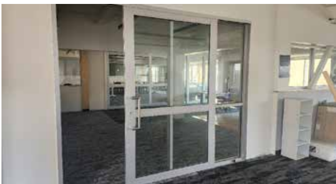
Installation of glass partition doors between 12B & Zone Room
